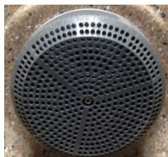
Keep the **SUCTION FITTINGS** (located in the foot well area) of the **ECO SPA** unobstructed and free from debris at all times.
